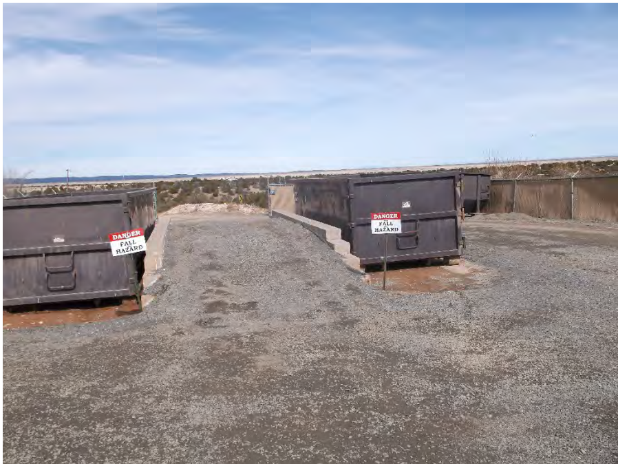
Elevated ramp between two roll off containers for waste disposal
