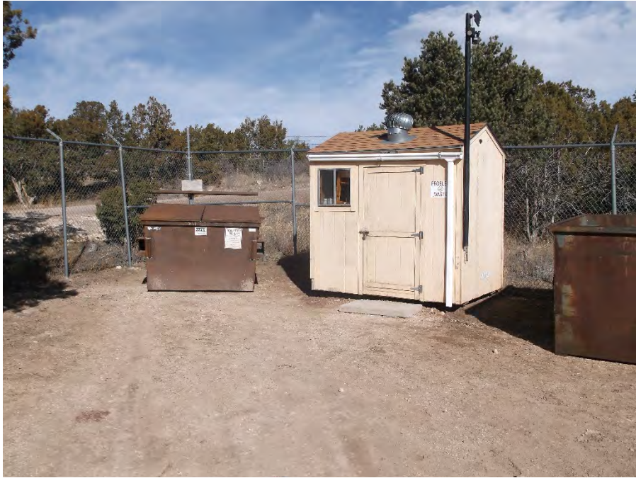
Ash Storage Bin and Attendant Shed
