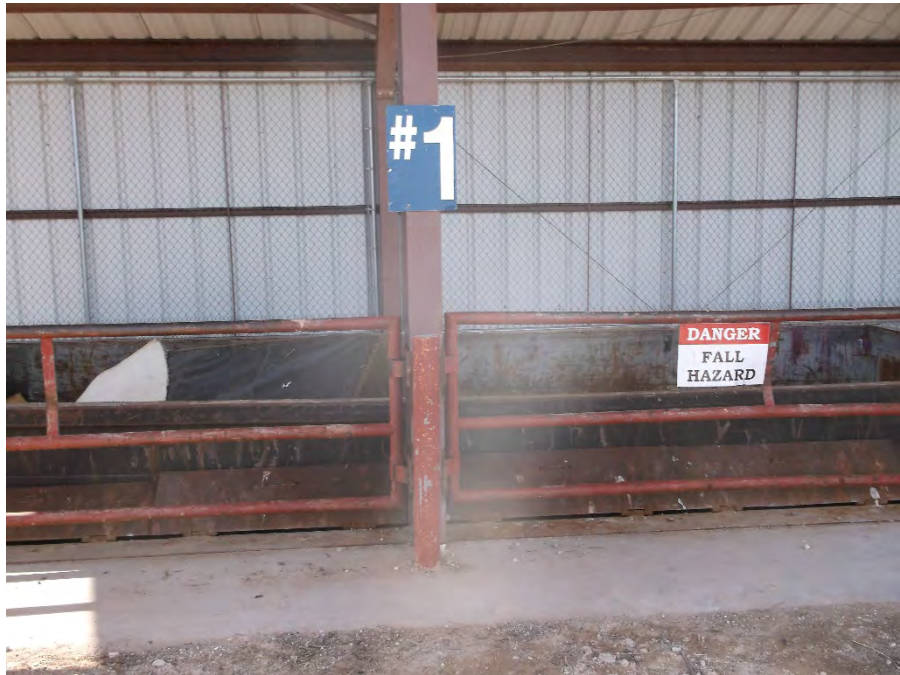
Two 40 yard Bulk Waste Disposal Bins
